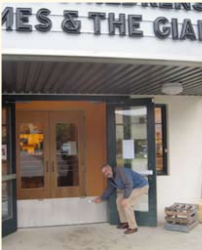
Theatre main entrance protected by FBS Vertical channels for Flood Barrier Shields were mounted during construction in 2006 onto door frames at the theatre's five doorways, including the 8-foot span at the main entrance shown here. The custom-made aluminum panels were easily and quickly inserted in the channels as Hurricane Irene approached in 2011, providing a virtually watertight barrier that protected the building's interior. Above, Architect Chip Greenberg points to the high-water mark of Irene's floodwaters.
