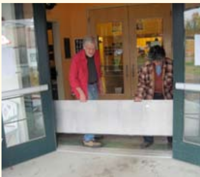
Inserting Flood Barrier Shield into the pre-installed tracks Bari Shamas (at right), president of the Board of Trustees for the New England Youth Theatre, inserts Flood Barrier Shield panels into pre-installed channels, with an assist from Associate Technical Director Jerry Stockman.
