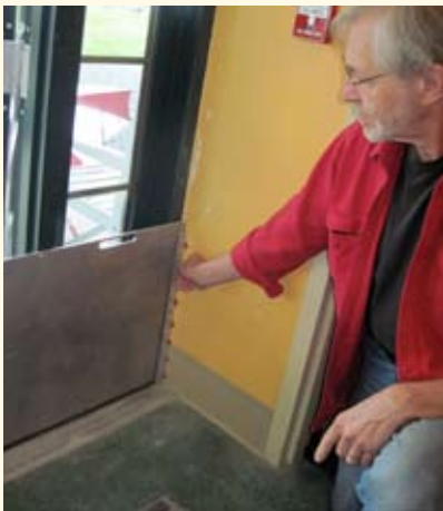
Securing Flood Barrier Shield in place Associate Technical Director Jerry Stockman tightens a set of thumbscrews to seal the Flood Barrier Shield panel against neoprene gaskets lining the installation channel. To accommodate the theatre's out-swinging doors, the channels were pre-installed on the interior of the door frame.
