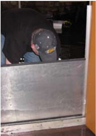
FBS protection in place A Flood Barrier Shield installed in this doorway of a Midwest home protected the interior of the house when floodwater in the garage rose to a height of 2 feet above the threshold.
